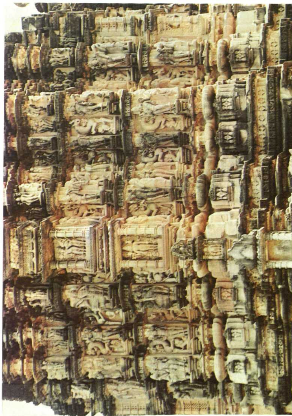
Devijagadambi Temple, Khajuraho : sanctum façade, affected by cryptogams, before chemical treatment
