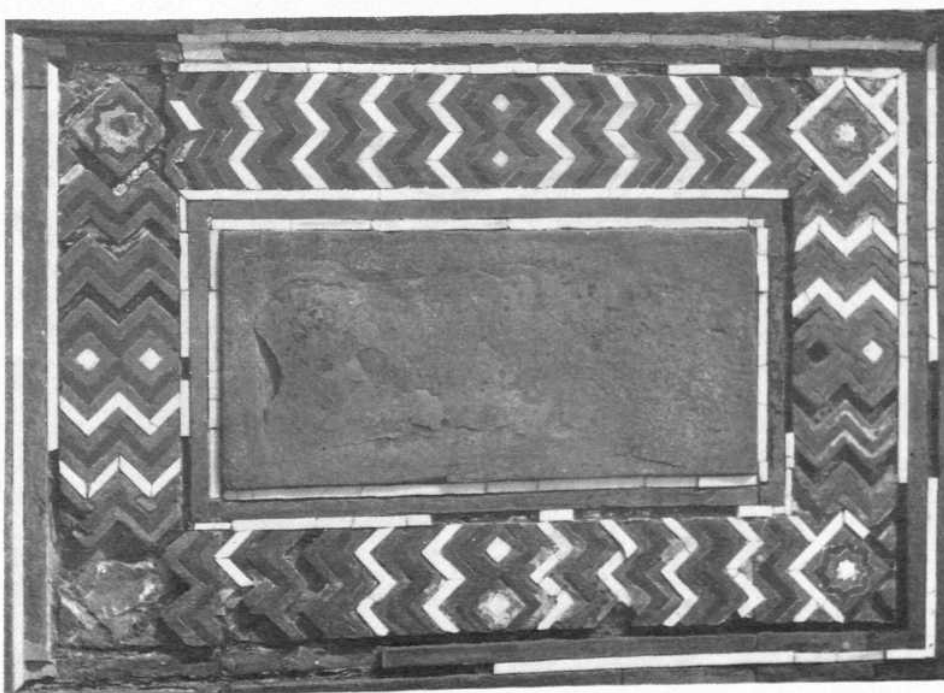
Agra: Taj Mahal, A, before and B, after restoration of missing inlay pieces of main gate. See p. 156
