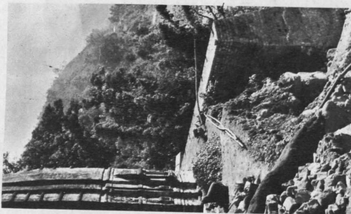
Trilokinath temple, Mandi: retaining wall, A, during, and B, after reconstruction. See p. 166
