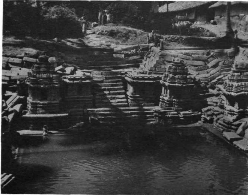
114 Hulikera : View showing the western wing of Kalyani before conservation. See page 214
