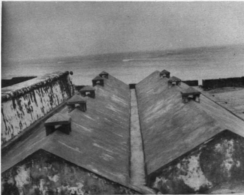
137 Fort St. Angelo, Cannanore : Showing the leaky terrace of the horse stables after conservation See page 223
