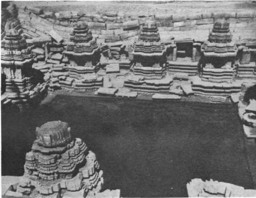
112 Hulikera : View showing the northern Wing of Kalyani before conservation. See page 214
