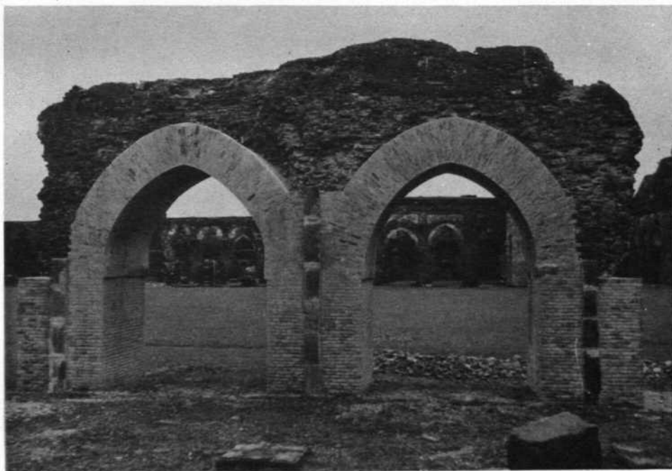
109 Adina : Two arches inside Adina Mosque in east after conservation. See page 210
