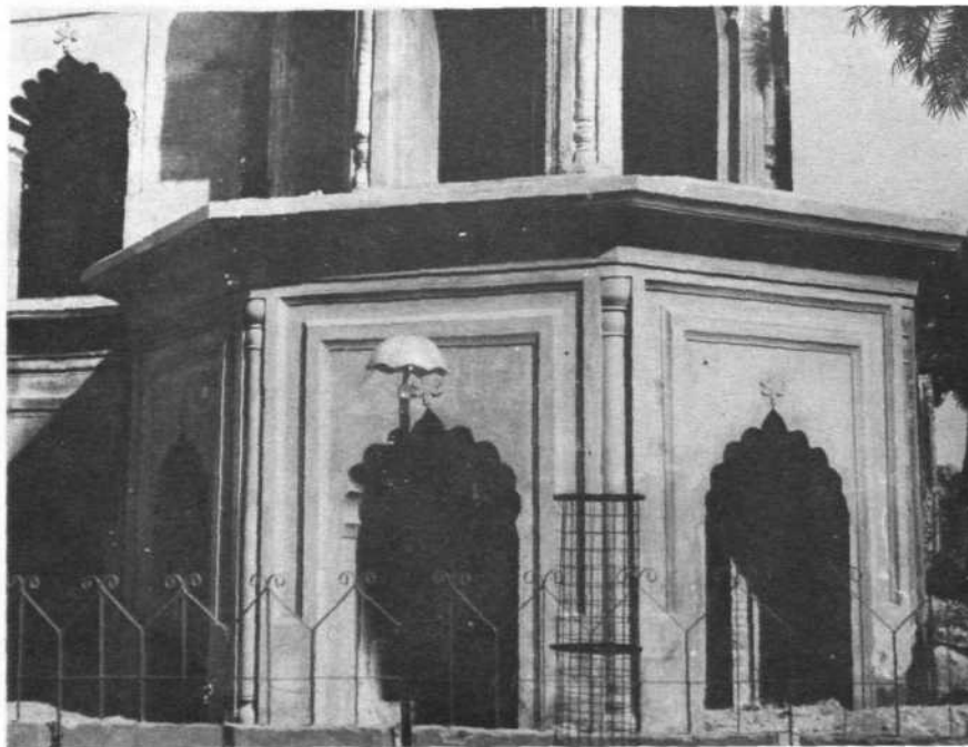
127 Lucknow Rumi Darwaja : South Bastion western facade after conservation. See page 219
