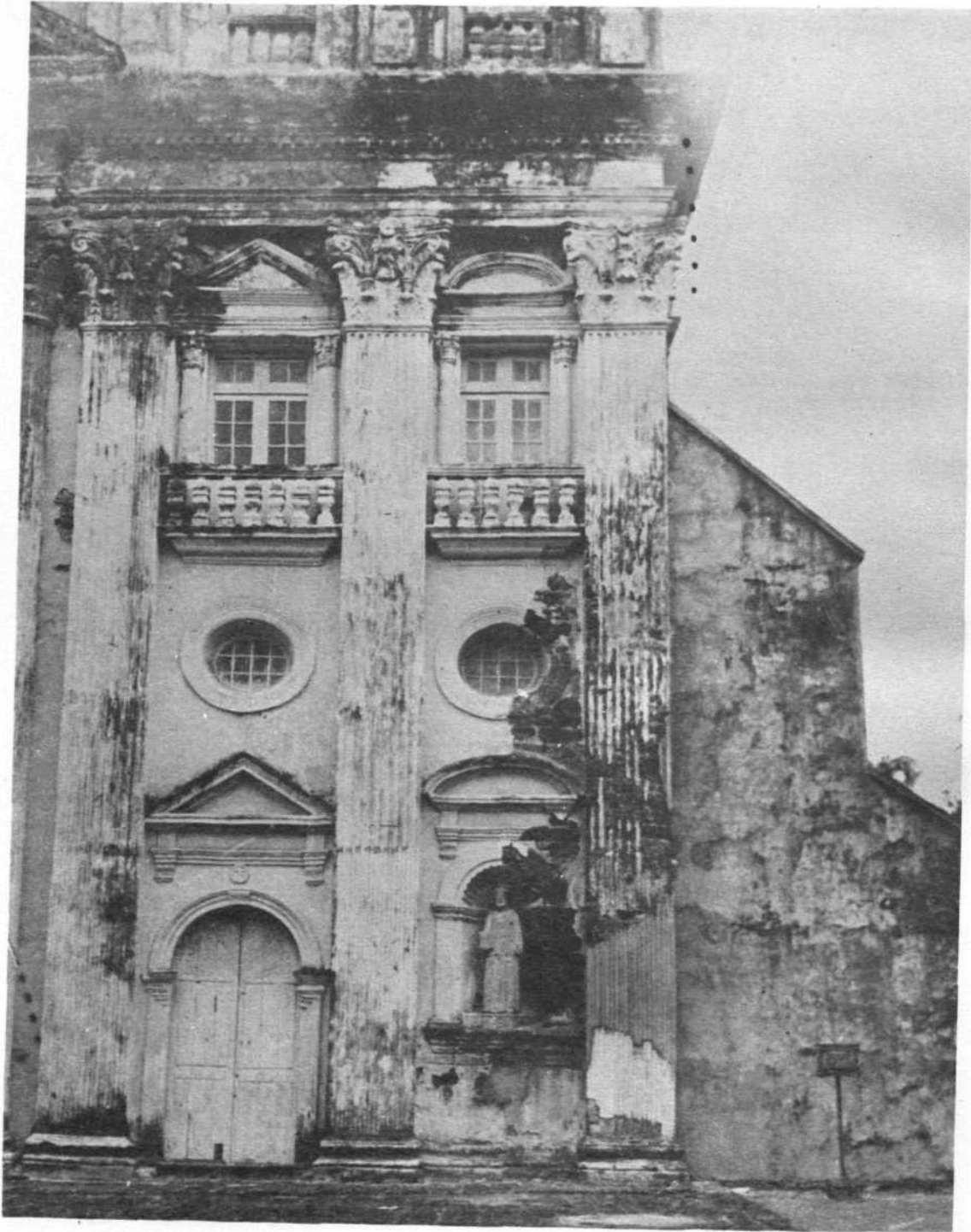
162 St. Cajethan Church : Close up of the part of facade from west before conservation. See page 227
