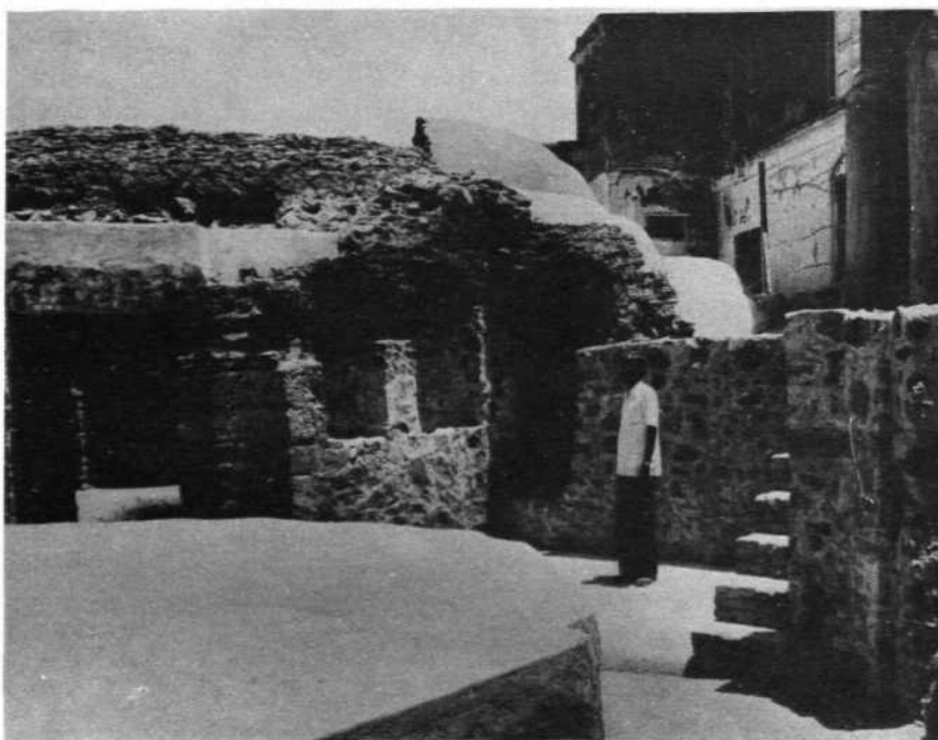
99 Burhanpur : Close-up view of Hammam after conservation. See page 206
