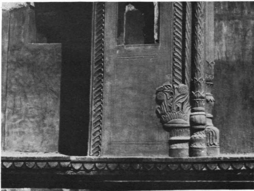
125 Asaf-uDaula's Imambara, Lucknow : Southern facade of 1st entrance gateway after conservation. See page 218
